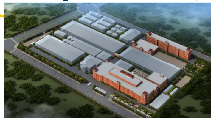
JiangSu- WuXi Site II (2007~)
